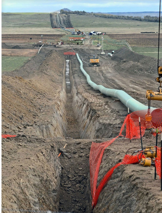
Dakota Access Pipeline
